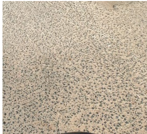
Gambar 13 Agregat Licin
