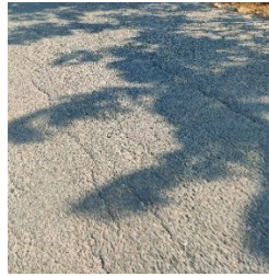
Gambar 8 Retak Diagonal
