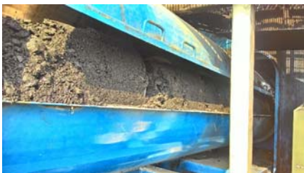
Gbr. 5 Screw Overload
