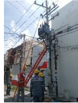
Figure 3. Fuse Cut Out (FCO) Termination
