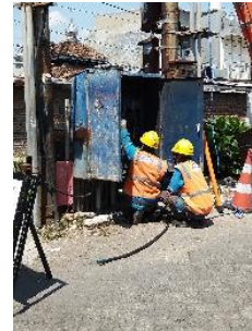
Figure 2. Voltage and Current Measurement Before Starting Maintenance
