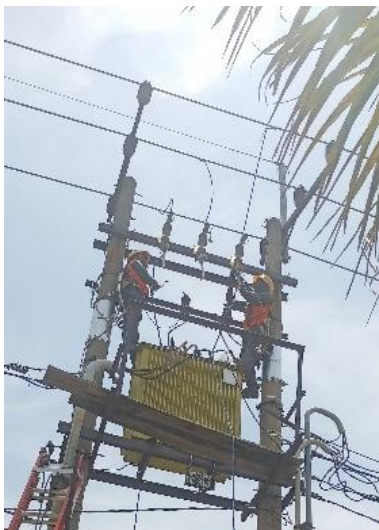
Figure 2. The Lightning Arrester replacement work was carried out by the HAR-C team PT. PLN (Persero) ULP Ngagel
