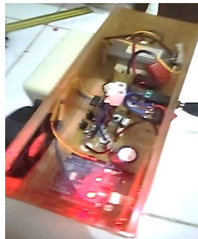
Figure 9. Inverter Realisation Image
