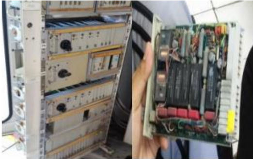
Figure 7 examinations and relay installation in PLGTU and GITET area
