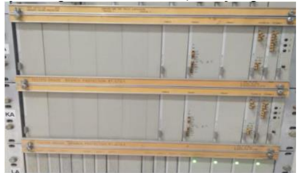
Figure 3. branch breaker failure
