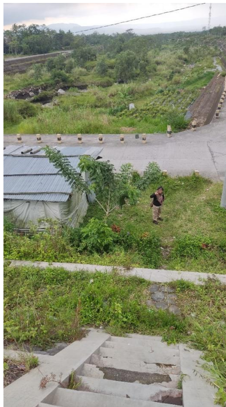
Figure 2. Photo of the Sabo Bronggang Dam Location. Source: Sony Eka, 17 February 2023
