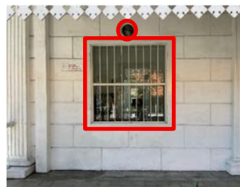
Figure 9. Window without shutters
