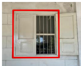
Figure 8. Window with shutters
