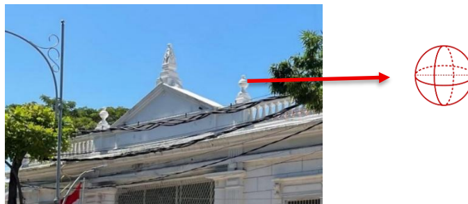
Figure 2. Building Roof Peak Ornaments
