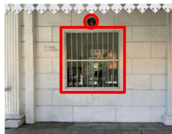
Figure 9. Window without shutters
